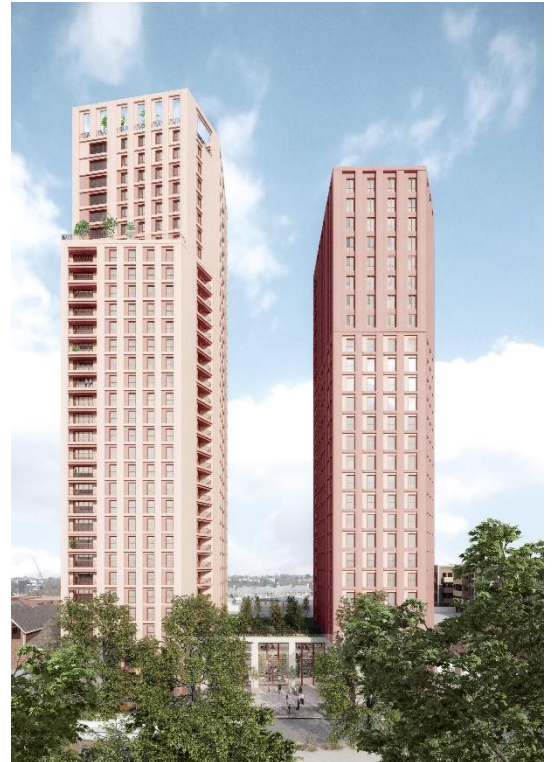
View from Selbourne Road
